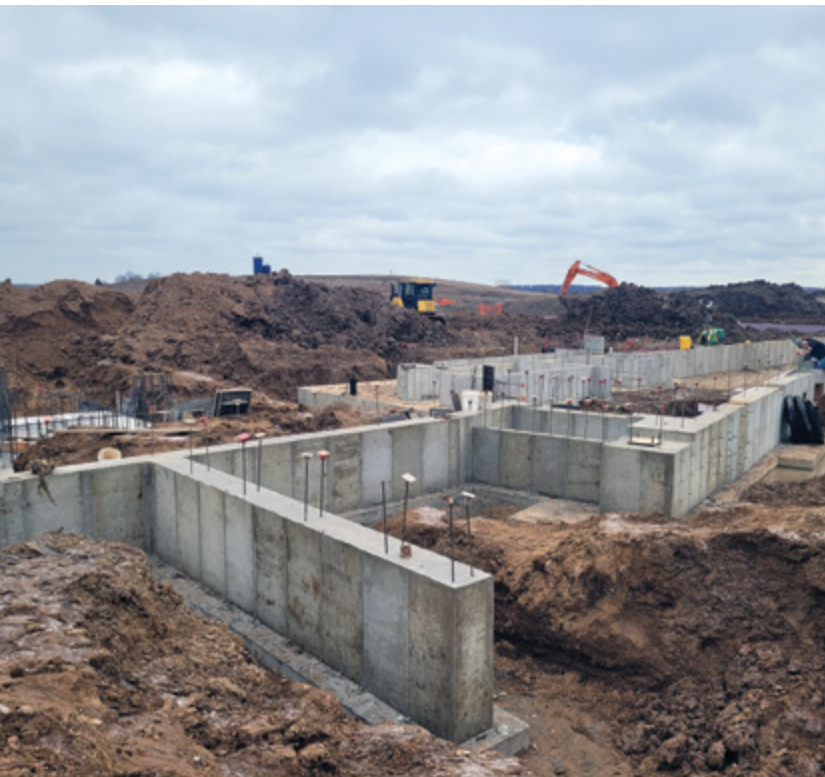
Construction of the Cal Community Center continues.
